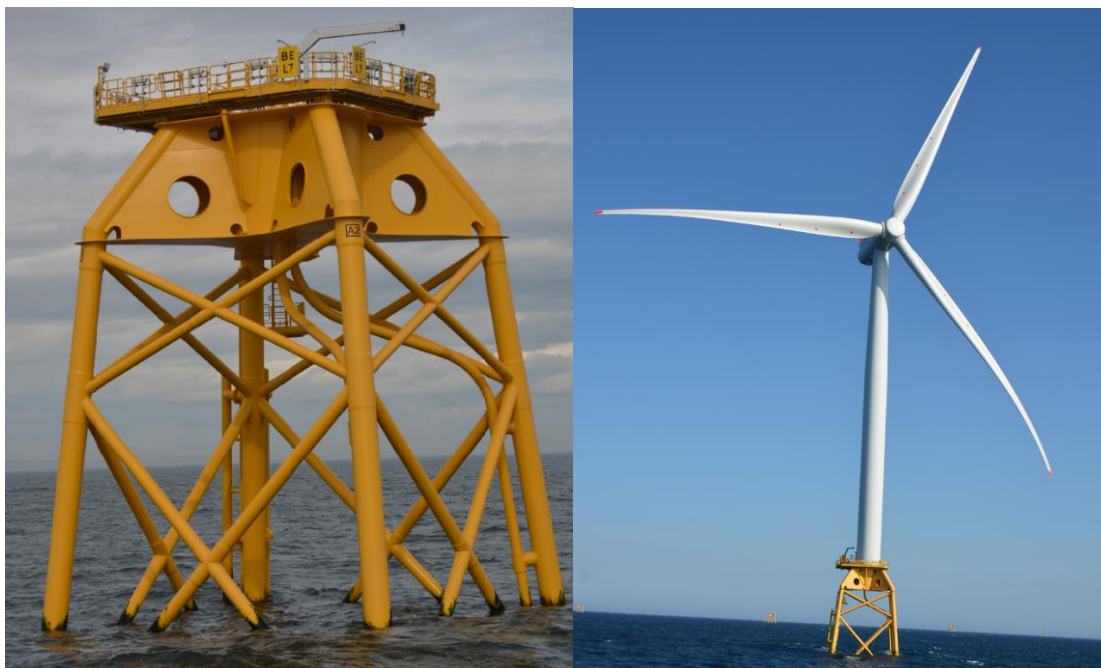
Fig 2. Foundation Jacket Pre and Post Installation of Turbine
