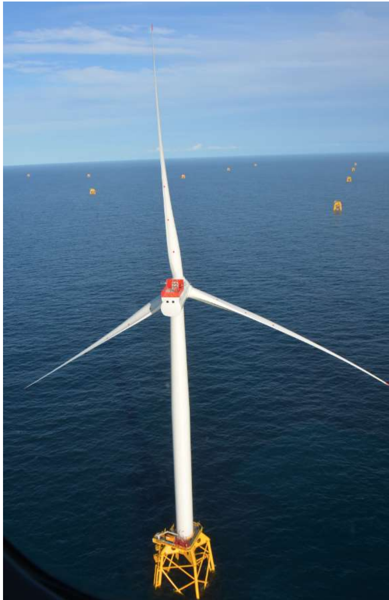
Fig. 5 Siemens SWT-7.0-154 WTG installed at Beatrice OWF
