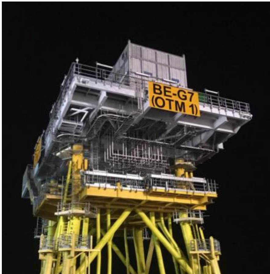
Fig 2 OTM 1 showing lower cable deck and J-tubes
