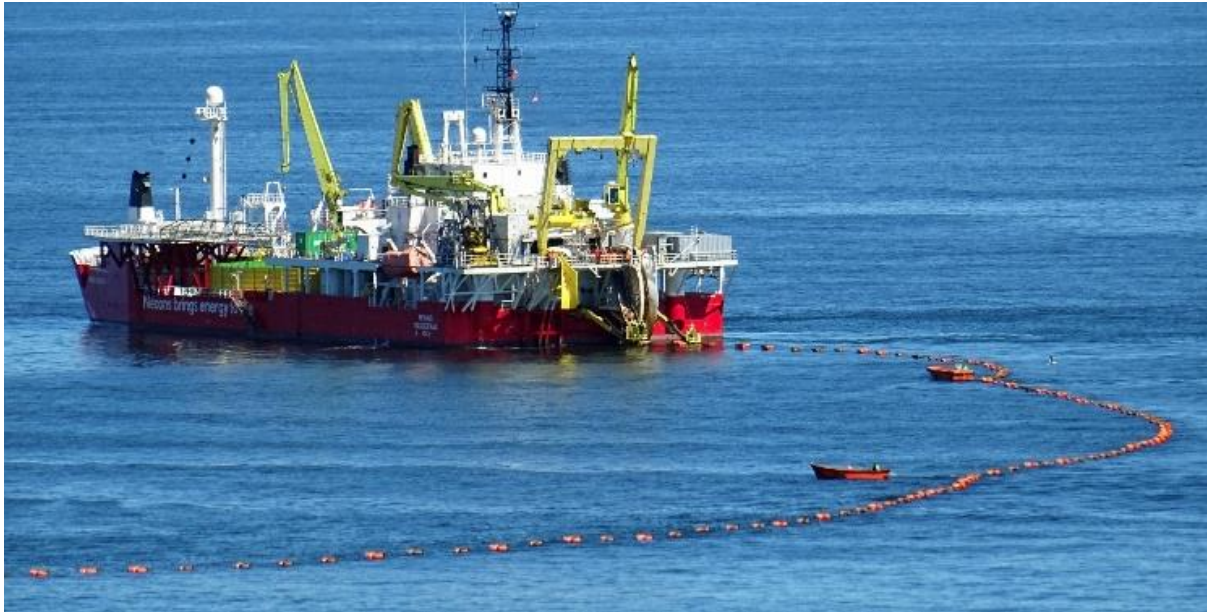
Fig 3 Cable being floated ashore from CLV Skagerrak
