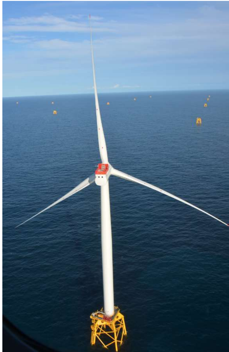
Fig. 5 Siemens SWT-7.0-154 WTG installed at Beatrice OWF
