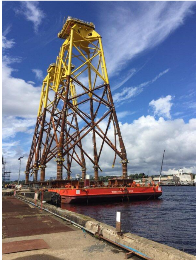
Fig.12 Jackets are transported in the vertical position secured on a cargo barge ready for installation.
