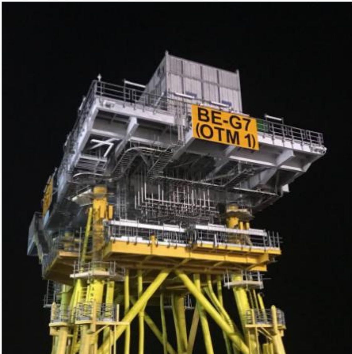
Fig 2 OTM 1 showing lower cable deck and J-tubes
